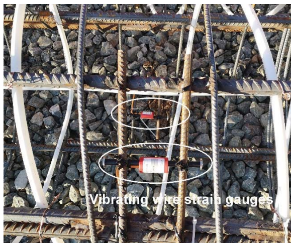
Fig. 10 A section from energy pile with installed vibrating wire sensors
