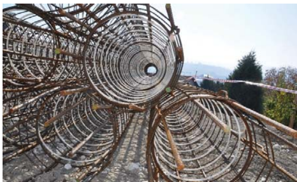
Fig. 5 Spiral shape pipes configuration installed in the 1000 mm piles
