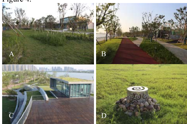
Figure 4. Early construction pictures of Yaojiang North Riverfront green open space. (A: Grass swales; B: Permeable pavement; C: Green roofs; D: Overfall gap)
