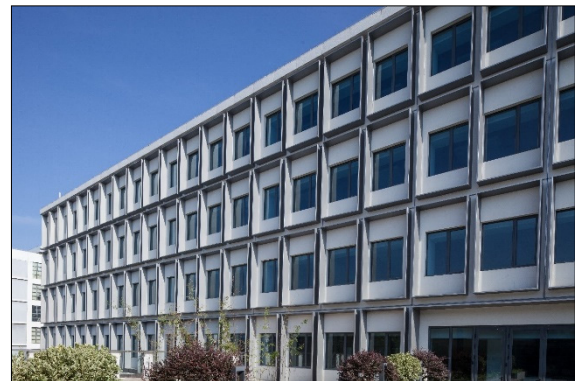
Fig 4. The prefabricated exterior wall
