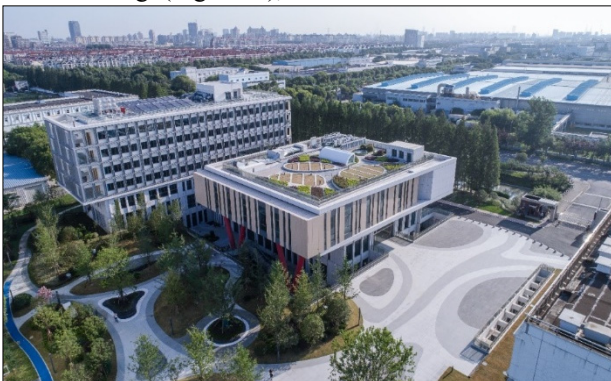
Fig 3. The bird view of the 10th building
