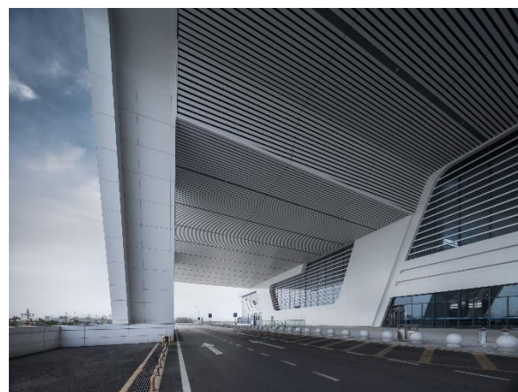
Figure 3: Rapid ramp in the square in front of the station
