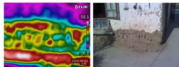
Fig8. Thermal imaging judgment of Building 2 disease
