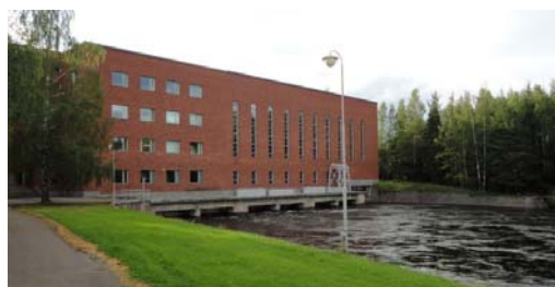
Fig. 7. Mankala Power Station along the Kymi River in Iitti, Finland [43]
