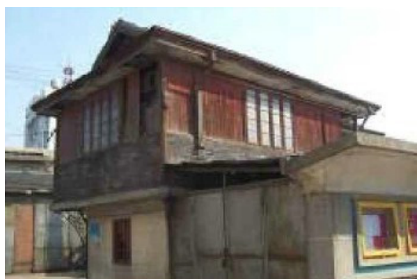
Figure 4. Office building of Zhenjiang Water Treatment Plant
