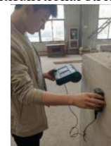
(a) Locating steel bars
