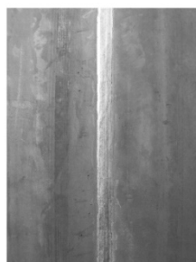
Figure 2. Grayscale image of welding seam
