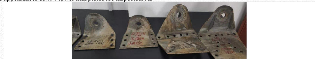
Figure 3. Deformed link plates of right cross arm of # 94 Tower.
