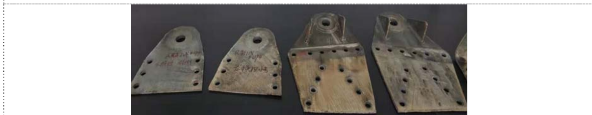
Figure 4. Undeformed link plates of the left cross arm of # 94 Tower.
