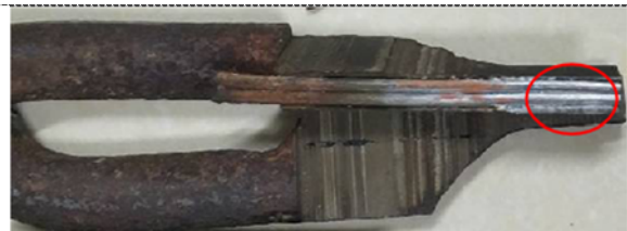
Figure 4. The steel core in the compression zone is not corroded.
