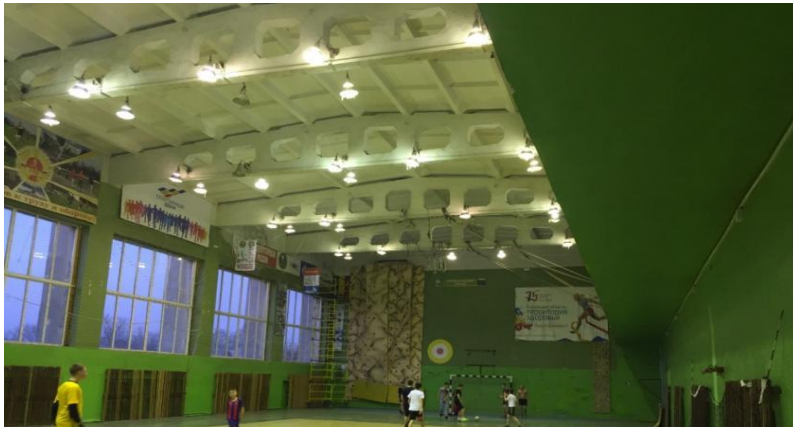
Fig. 8. School game hall with load-bearing structures made of precast concrete structures.
