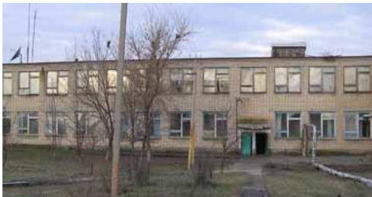
Fig. 9. Facade of the school building in the village of Karachevsky
