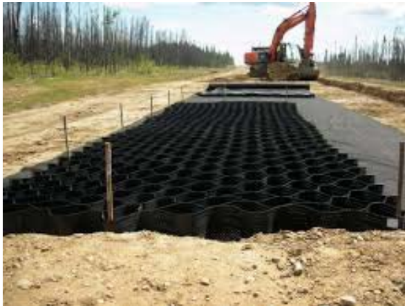
Fig. 1. Environmental-friendly geogrid in road construction.
