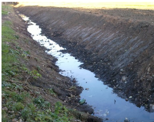
Fig. 2. Reclamation canal in the process of cleaning and renewal
