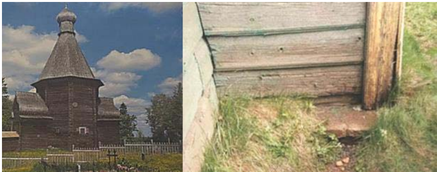
Fig. 4. Biological deterioration of the enclosure of Nikol'skaya Church. Archangel'sk Region, Lyavlya Village.
