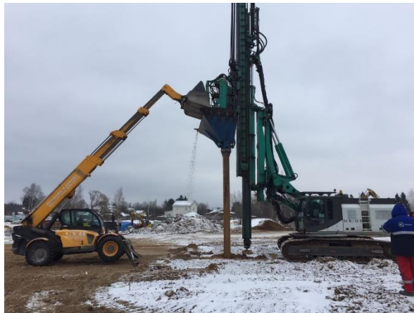
Fig. 7. General view of the equipment for installation of vibro stone columns.
