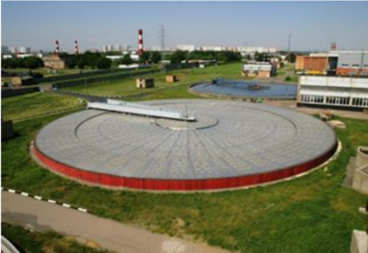
Fig. 2. Example of a floating flooring at a primary sedimentation tank
