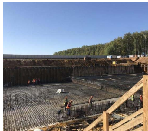
Fig. 5. Construction of waste-recycling plant
