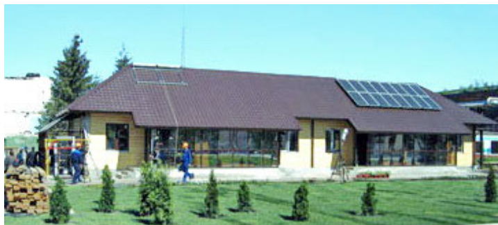
Fig 1. Energy-efficient house in the territory of the Technopolis «Himgrad» Kazan city, Vosstaniya st., 100.
