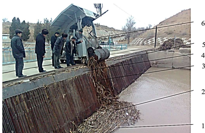
Fig. 1. The process of removing debris collected in front of the grate at the pump station Amu-Bukhara-1: 1 – mouth; 2 – grid holding traps; 3 – streams falling back into channel; 4 – car moving rails; 5 – dryer cover; 6 – the machine that moves the cleaning device.
