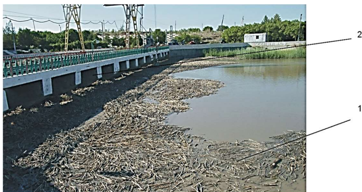
Fig. 2. Collection of effluents in front of the grate at the Amu-Bukhara-2 pumping station: 1 – mineral and organic particles; 2 – water access paths to the forechamber.
