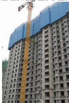
Fig. 2 Prefabricated Project - 7# Building of Red Fort Lan Palace
