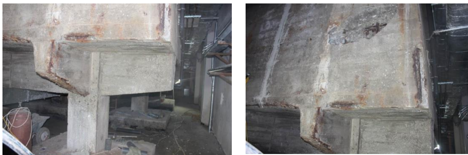
Fig. 1 and 2. General view of the pool bowl structure.
