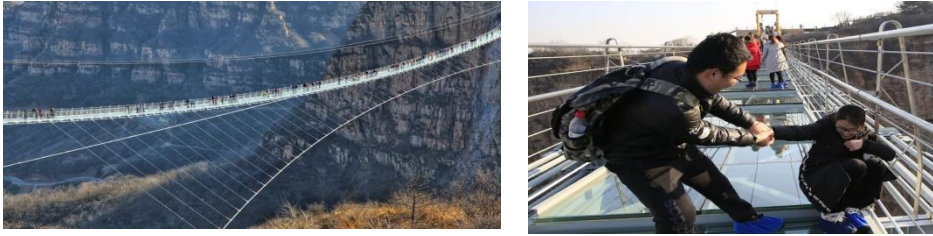
Fig. 2. Hongyagu Bridge, China.
