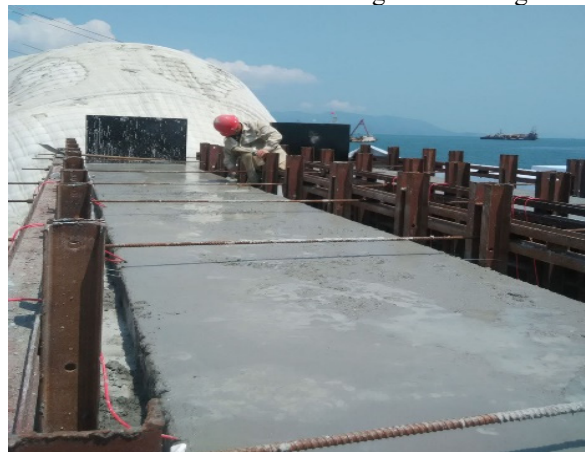
Fig. 5 Two mass concrete test blocks have been poured
