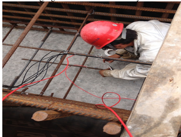
Fig. 4 Installation of test block concrete strain gauge
