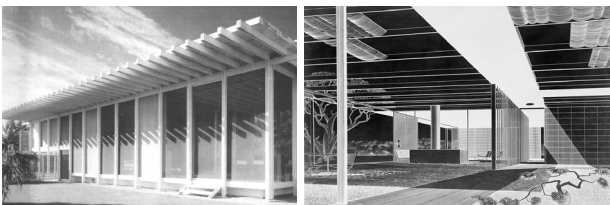
Fig. 7. Harkavy Residence Fig. 8. Watson Residence
