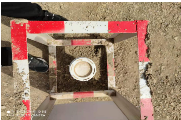
Picture 3 Settlement detection device
