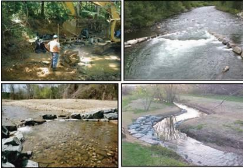
Fig. 1. River restoration projects are undertaken to enhance habitat heterogeneity. Top left: Large equipment often used to reconfigure and create artificial pools and habitat structures. Top right: Rocks placed in the channel can deflect flow to increase variable habitat. Bottom right: Artificial meanders created by reconfiguring the channel. Bottom left: Inflow rock structures can create shallow pools downstream [1].
