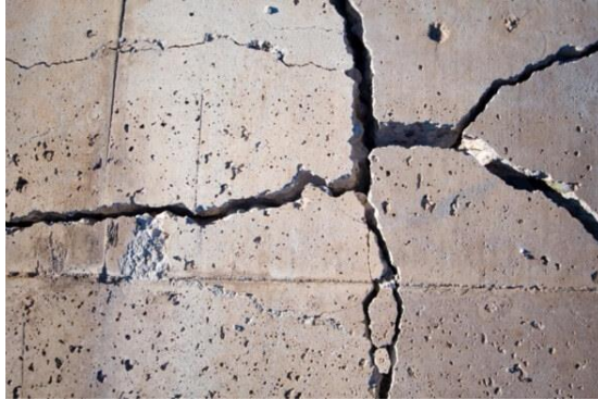
Fig. 3. Deformation of concrete along the length of the reinforcing bars.
