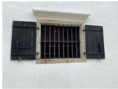
Fig. 4. The wood window of Casa da Cheang.
