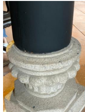
Fig. 6. The column foundation of Casa da Cheang.
