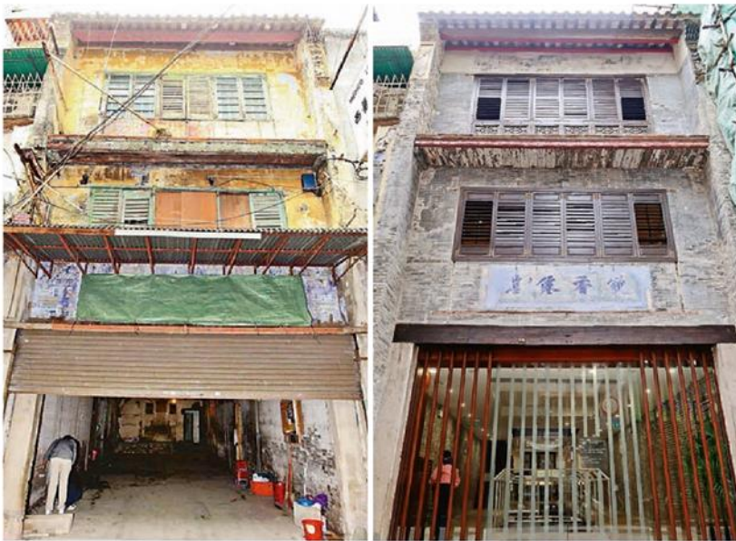
Fig. 3. Comparison of Chong Sai Pharmacy before and after restoration (left old and right new).
