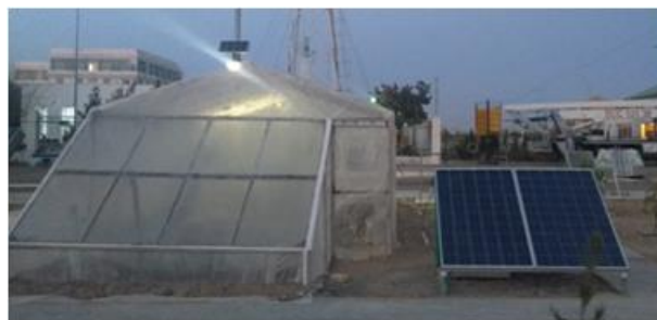
Fig. 2. General appearance of the helium greenhouse.
