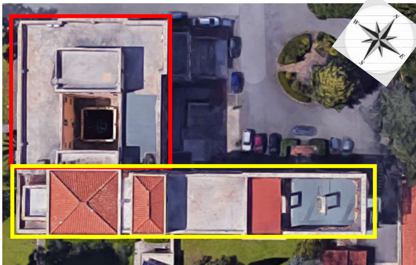
Fig. 1. Aerial picture of the reference building
