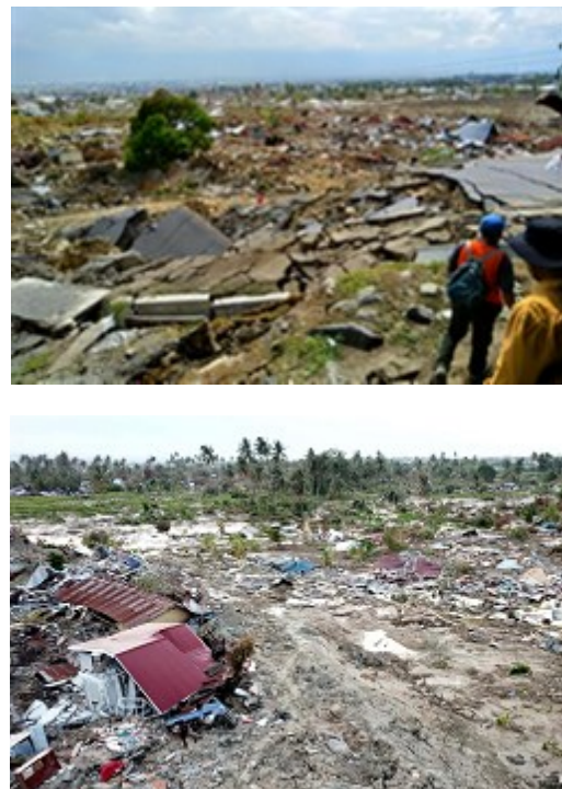
Fig. 1. Flow liquefaction disaster phenomena in Balaroa (above), and Petobo areas (below) due to the 28 September 2018 earthquake ( M_w 7.5).
