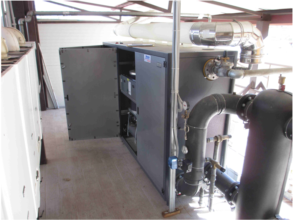
Fig. 6. Modular heat generator supplied complete with a containment cabinet and a hydraulic separator.
