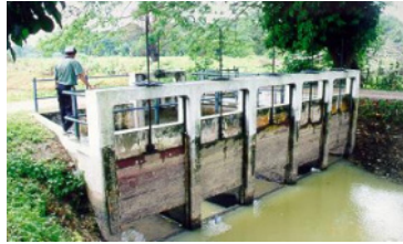
Fig. 2. Chamber with rectangular box-typed inlet controlled by sluice gates.
