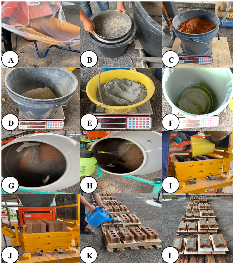
Fig. 2. Interlocking hollow clay block production a) Crushing of laterite soil; b) Sieving of sand; c) Weighing of laterite soil; d) Weighing of sand; e) Weighing of cement; f) Weighing of water; g) Dry mixing of soil, sand and cement; h) Addition of water; i) Pouring mixture into mould; j) Mixture compression; k) Watering the IHBS; l) Curing of IHBS
