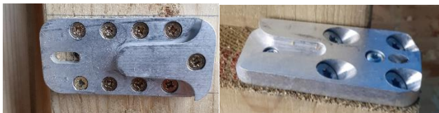
Fig. 1 Connector to enable the dismantling of the wooden structure (0,14kg aluminium + 0,78kg galvanised steel screws per connector). One connector is needed for each 38x100mm beam connection, two connectors are needed for each 38x200 mm beam connection.
