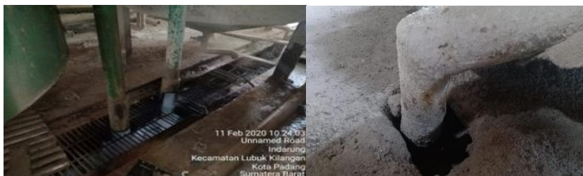
Fig. 5. Changes brought by the water efficiency program before (left) and after (right) the valve has been closed in the Indarung 2/3 factory water channel
