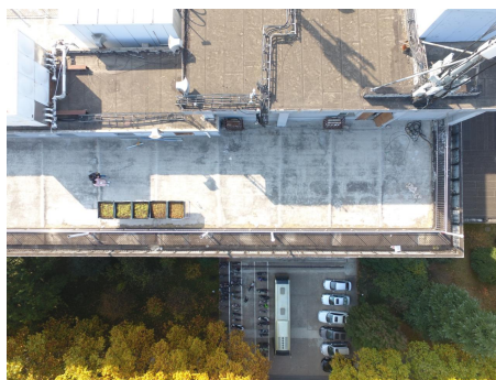
Fig. 2. Roof greening air purification test
