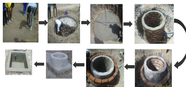
Figure 29 : Construction of an experimental cylindrical biodigester unit using dead neem leaves [32]
