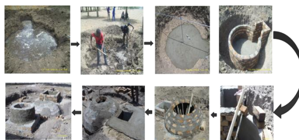
Figure 30: Construction of an experimental fixed dome biodigester unit using dead neem leaves ([32])
