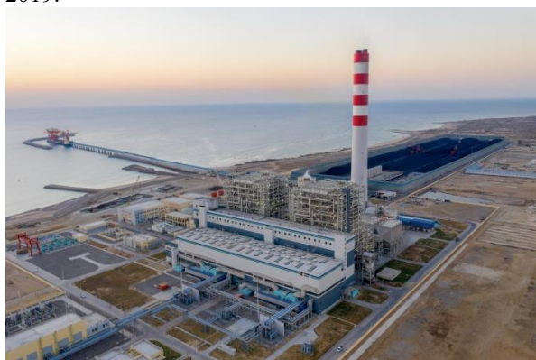
Fig. 1. Aerial view of the 2×660MW coal-fired power project.
