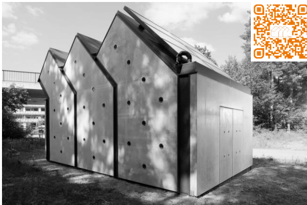
Figure 2: Full-scale demonstrator 'SmallHouse IV' from the southwest made of multifunctional building parts, incl. two exchangeable elements and the solar thermal collector.
