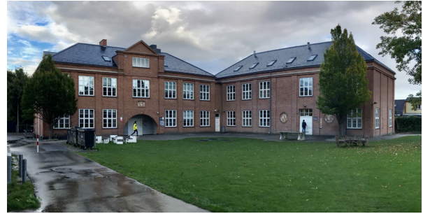
Figure 1: Photo of the building in question.
