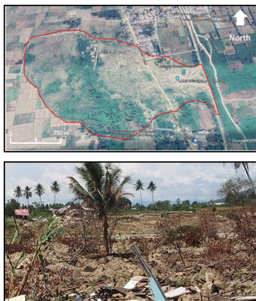
Fig. 1. The areal photograph of the Sibalaya flow liquefaction (top) and destroyed houses (bottom).
