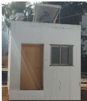
Fig. 1. View of the cubicle
