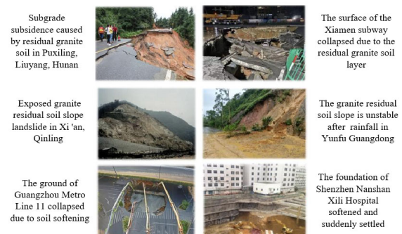
Fig. 1 Geological hazards of unsaturated granite residual soil [2]
