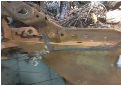
Fig. 3. A part of battery wiring on the side of the terminal post (+).
