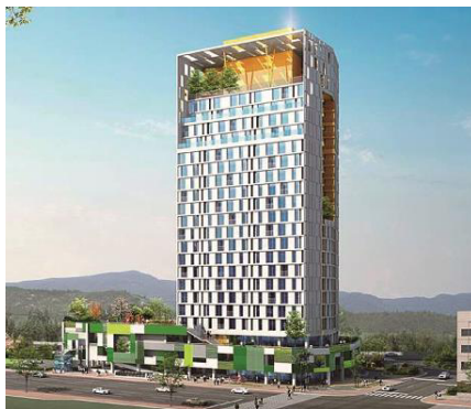
Fig. 1. Picture of analysis building.
