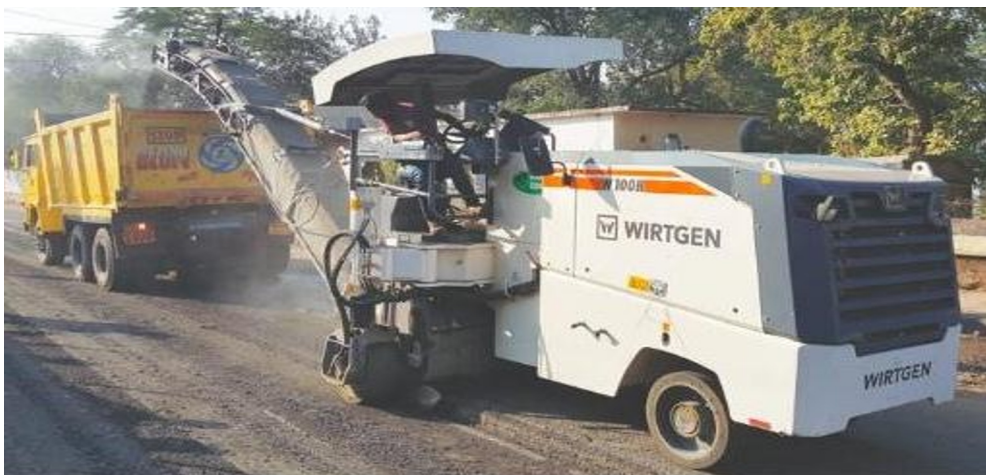
Fig. 1. Milling Machine for RAP extraction from Old Pavement
