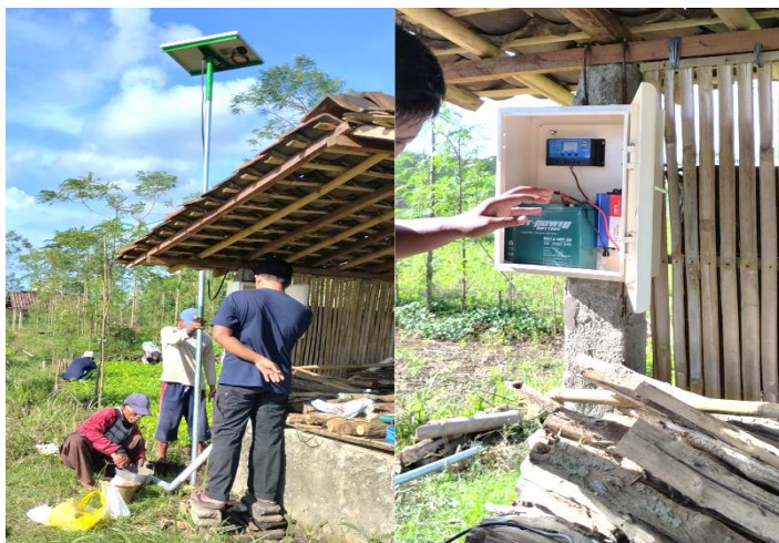
Fig. 4. Installation of the solar-powered hut (Pragak village).
